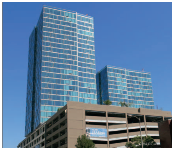
'The Vermont' is a Studrail® project located in Los Angeles, CA. It was completed in 2013.
