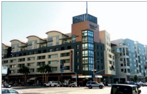
'Wilshire La Brea Apartments' is a Studrail® project located in Los Angeles CA. It was completed in 2012.
