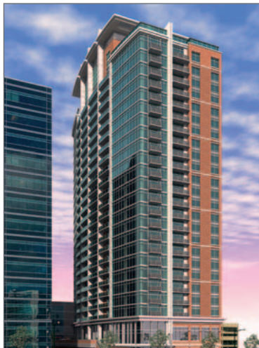
'Centergy North' is a Studrail® project in Atlanta GA, that began construction in 2014.
